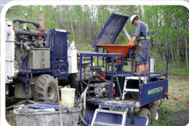
MOBILE GROUT PLANT - IN USE
